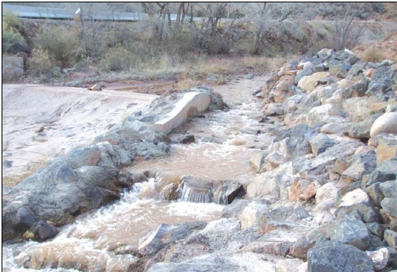
This diversion, however, constituted a barrier to upstream fish movement. The fish could not easily move out of the Virgin River into La Verkin Creek. The Program, the District and the Wilson family collaborated in order to come up with a win-win situation whereby both irrigation needs and fish needs were met.
