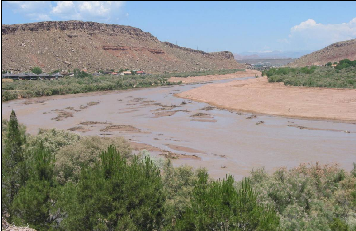
Figure 19 Over-widened channel excavations
