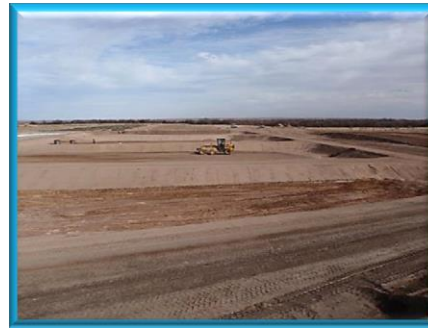
C-SERIES POND CONSTRUCTION, USFWS PHOTO
